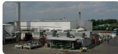
Roeselare: Hazardous waste
