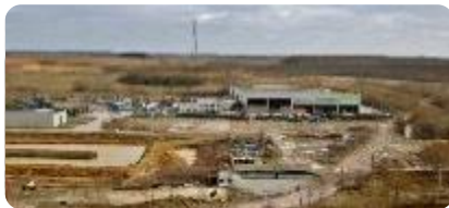
Mont-Saint-Guibert: Commercial Waste collection and sorting line
