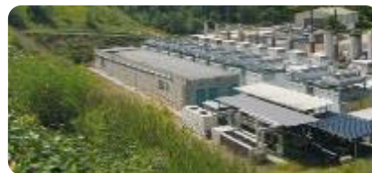
CETEM: landfill with green power
