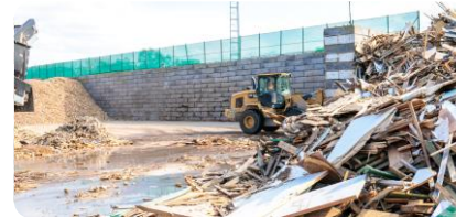
Kampenhout: commercial waste collection and organic waste pre-treatment
